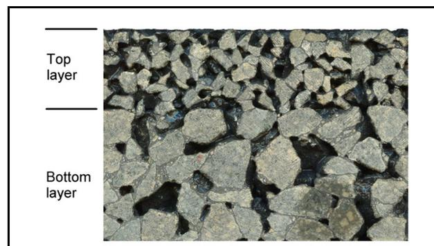
Figure 7: Structure of double-layered Porous Asphalt
