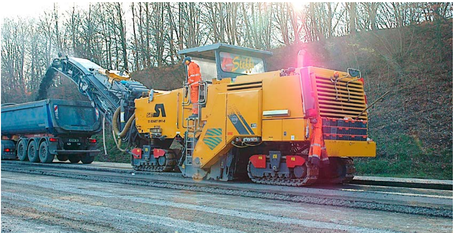
Figure 6. Milling of existing asphalt pavement
