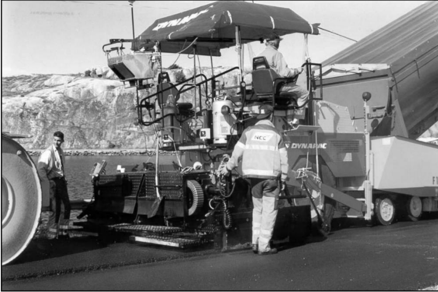
Figure 5. The temperature scanner mounted on the paver
