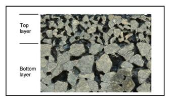
Figure 7: Structure of double- layered Porous Asphalt
