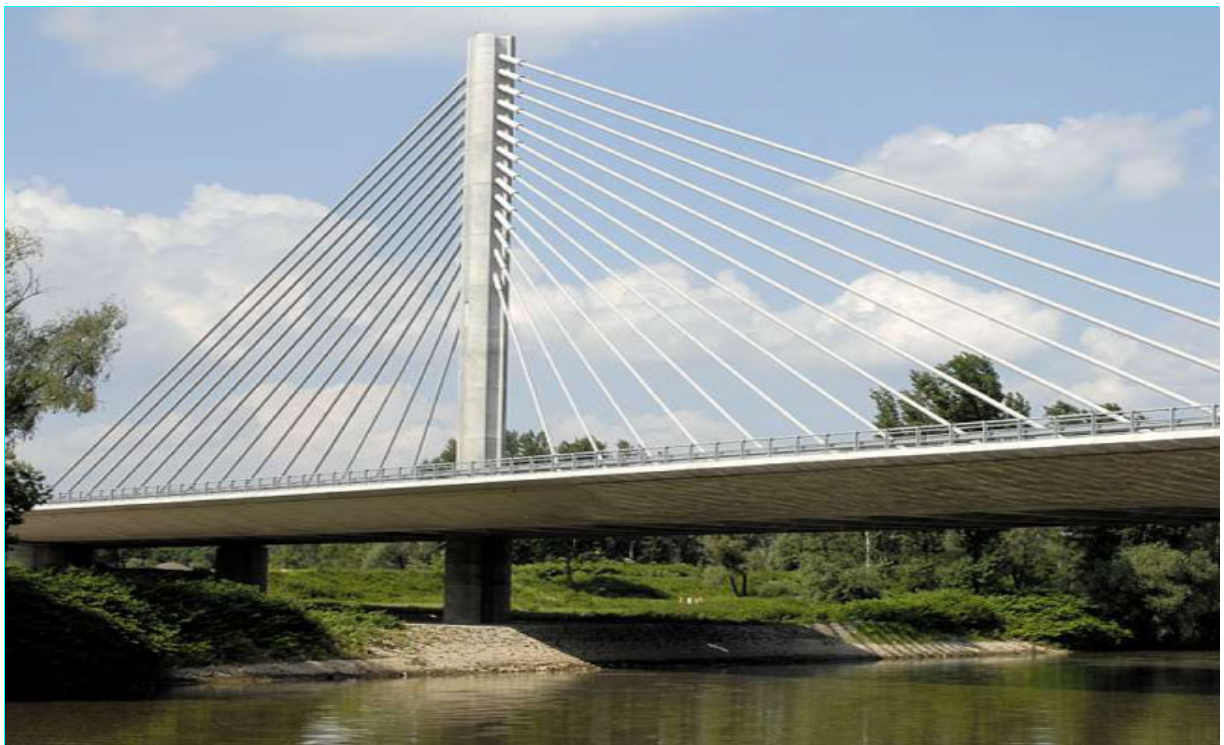
Bridge in motorway D 47 in Czech Republic on the river Odra (the length of the main span is 105 m)
