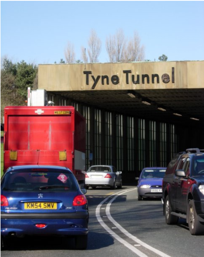
Tyne Tunnel approach
