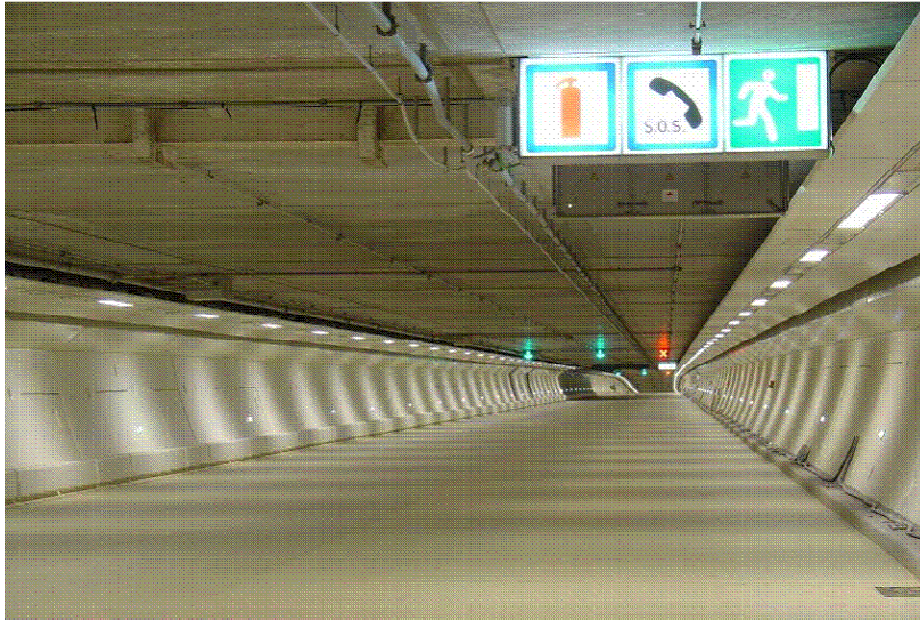
A-86 tunnel from Rueil Malmaison to A 13 motorway
