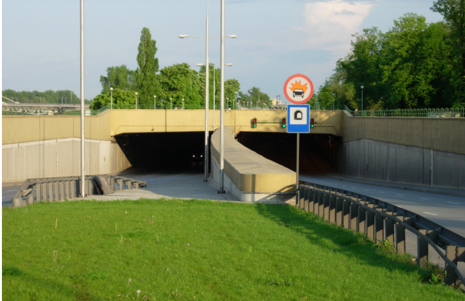
General view of northern in/out of the Wislostrada Tunnel
