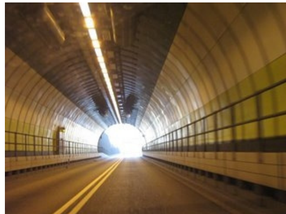
Dartford Tunnel interior
