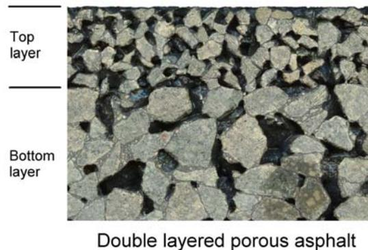
Figure 3.4. Double layered porous asphalt.
